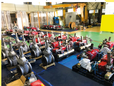
Valves undergoing inspection during customer's plant shutdown.
