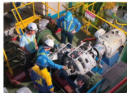
On-site inspection of pump in operation for signs of malfunction or abnormalities.
